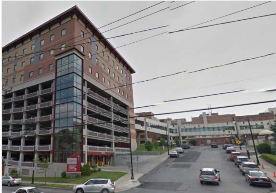
A Google street view image of the St. Joseph's Hospital Health Center in Syracuse, N.Y. (Credit: Google)
